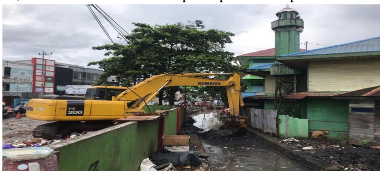
Fig 2. River dredging carried out by the Banjarmasin City Government
